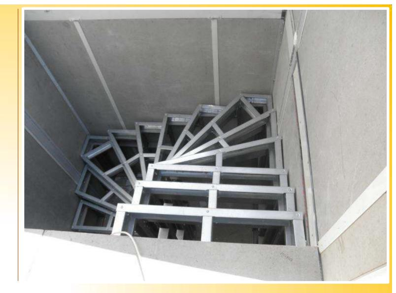
Staircase structure in lighsteel galvanized
