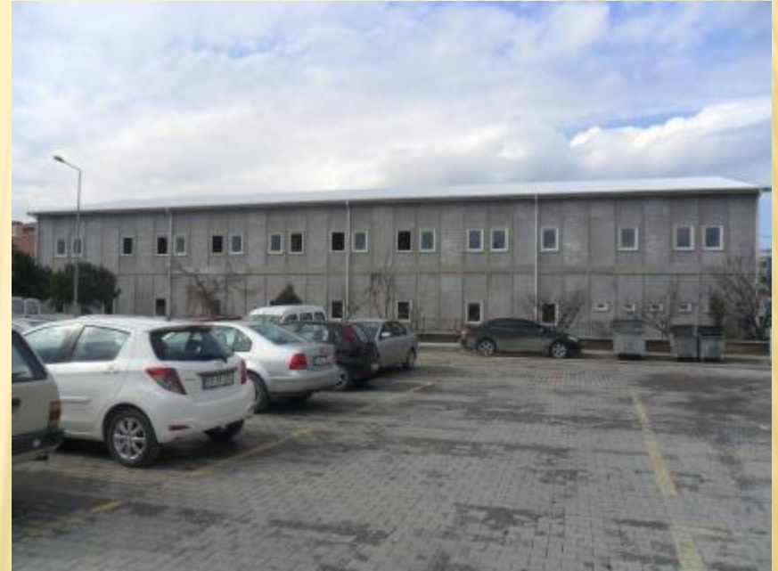
BUILDING COMPLETED (FOR PAINTING)
